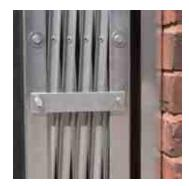
Retainer straps hold door gates in retracted position.
